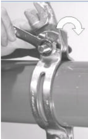
Tighten top and bottom nuts to proper torque, reference torque chart.
